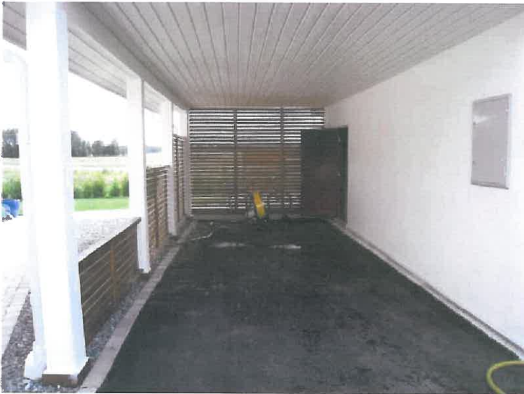
Picture 1: Entry from the carport.
